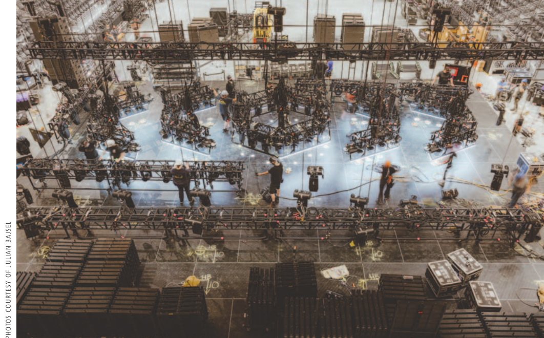
Figures 1A and 1B – Odesza's 2022 Last Goodbye tour used 53 Broadweigh shackles to publish real-time load cell data to a website for access by all departments as needed. Data logging also allowed daily review of the data. Left is the stage at the start of load-in; right is the truss structure in the process of being flown.
