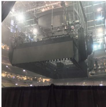
the load distribution of the mothergrid trusses need to be managed effectively without impeding on the speed of the load ins. One of the reasons we specify the BroadWeigh kit time and again is because all the load cells can travel within the trussing which make them much easier to handle at the beginning and end of each show.
